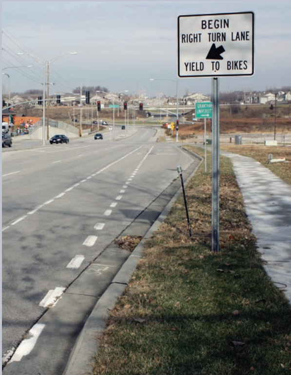
This bicycle lane and right turn merge on N. Congress Avenue in Kansas City, Mo., provides a facility for cyclists, while informing motorists how to safely merge right across the bike lane.
