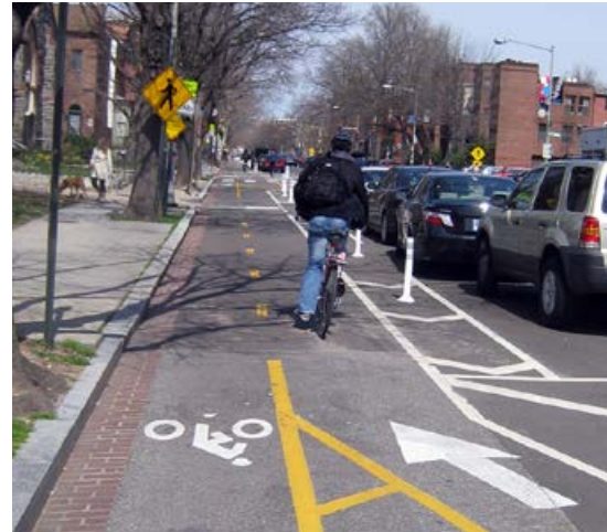
Figure 29 | Bike Lane —Protected / Cycle Track
