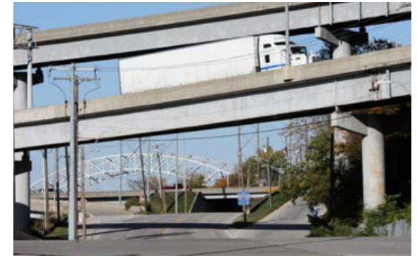
Figure 10 | Physical barriers can deter bicyclists.
