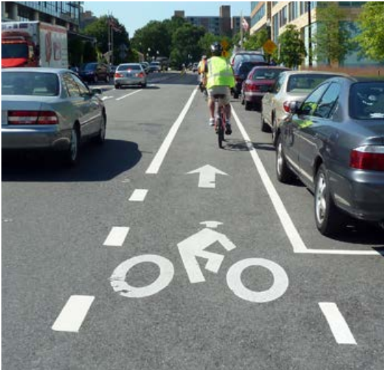
Figure 28 | Bike Lane — Buffered
