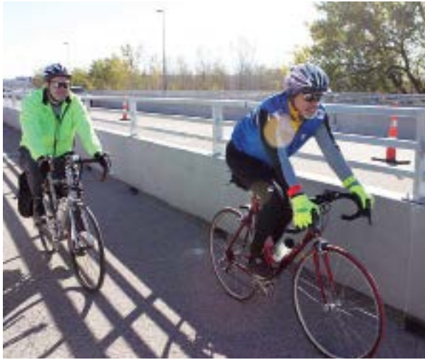
Figure 8 | The safest place for a bicyclist is in a designated bicycle facility like an on-road bike route, bike lane or separated bicycle-only path; the least safe is on a sidewalk. 11
