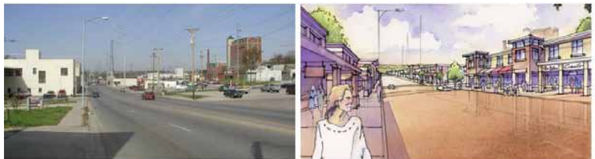
Leavenworth Street looking west from 39th Street (left). Concept rendering showing Leavenworth Street redevelopment based on design guidelines (right).
