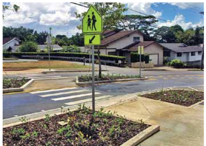
Angled crosswalks not only provide a safety refuge for pedestrians, but also encourages pedestrians to look for oncoming traffic before crossing the roadway. (Photo courtesy of EDAW)
