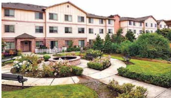
Alderwood Court Senior Apartments in Lynnwood, Wash., participates in a program that provides affordable rental apartment homes for senior residents. (Photo courtesy of EDAAW)
