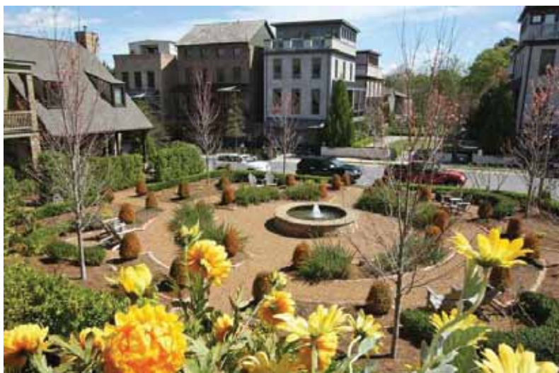
This high-density housing in Woodstock, Ga., combines part preservation, part new construction to create mixed-use structures that create a strong neighborhood character while respecting architectural tradition. (Photo courtesy of EDAW)
