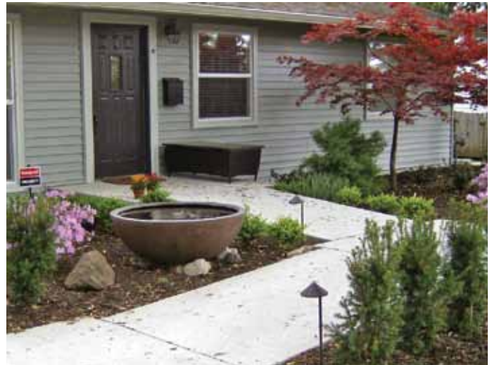
Accessible remodeling such as this sloping ramp from driveway to front door accommodates people through all life stages. (Photo used with the permission of KC MASS Services, Inc.)
