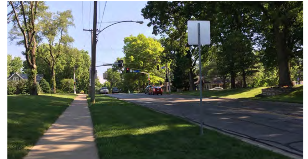
Mission Rd south of W 63rd St, looking north. Photo: NPS
