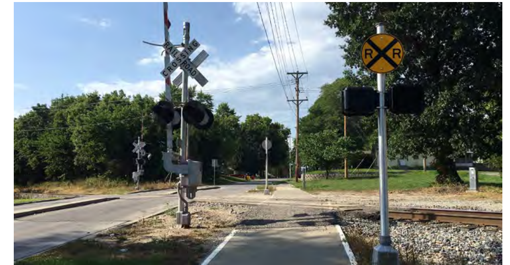
Signalized pedestrian crossing of railroad tracks on McCoy St looking north. Photo: NPS
