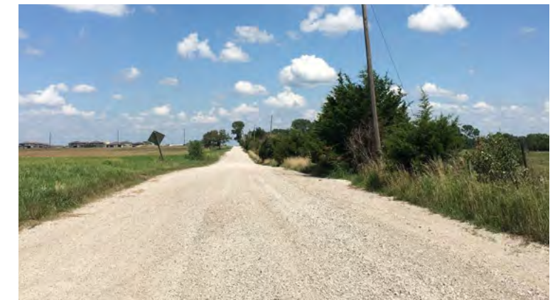
W 167th St west of road closure at US 169/KS-7, looking east. Photo: NPS
