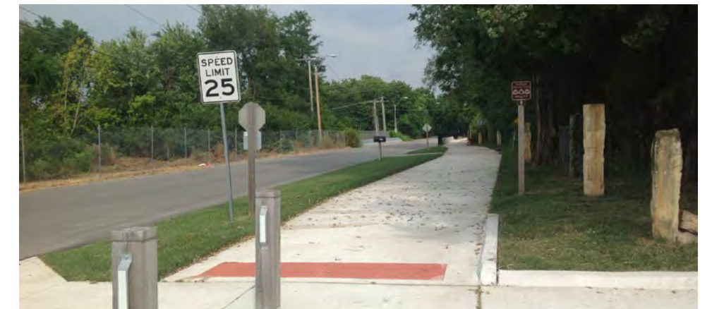
Trail along E 93rd St east of Schumacher Park, looking east. Photo: NPS
