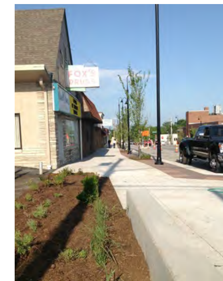
New streetscape on E 63rd St looking east. Photo NPS
