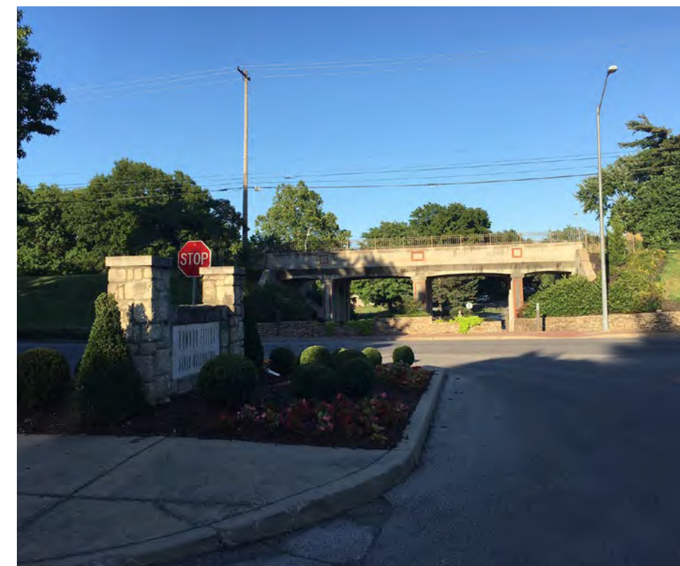
Trolley Track Trail bridge at Edgevale and Wornall Rds, looking southwest. Photo: NPS
