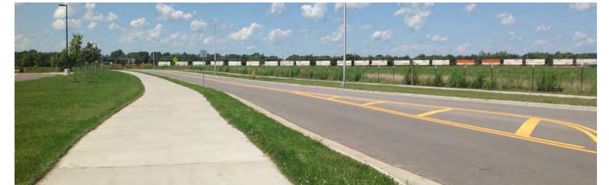
Side path in front of Trail Ridge Middle School on Grand St, looking west. Photo: NPS
