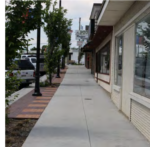
Streetscape improvements on E 63rd St, looking west.
