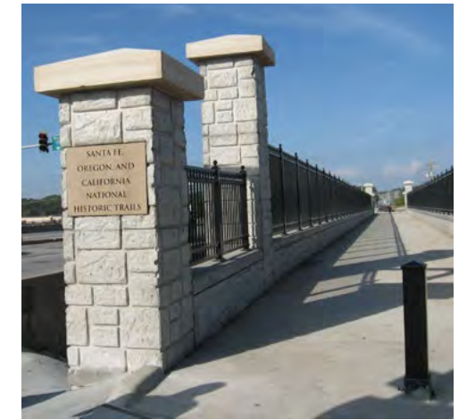
Powder Mill pedestrian bridge over I-435.
