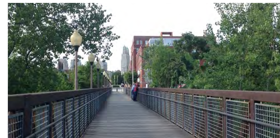
On the Town of Kansas Bridge, looking south. Photo: NPS
