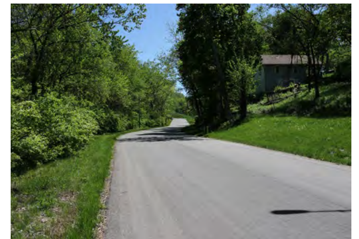
Mallinson Rd near Mallinson Elementary, looking east.
