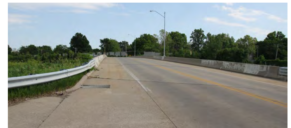
Bridge over I-435 on Grandview Rd, looking south. Photo: Vireo
