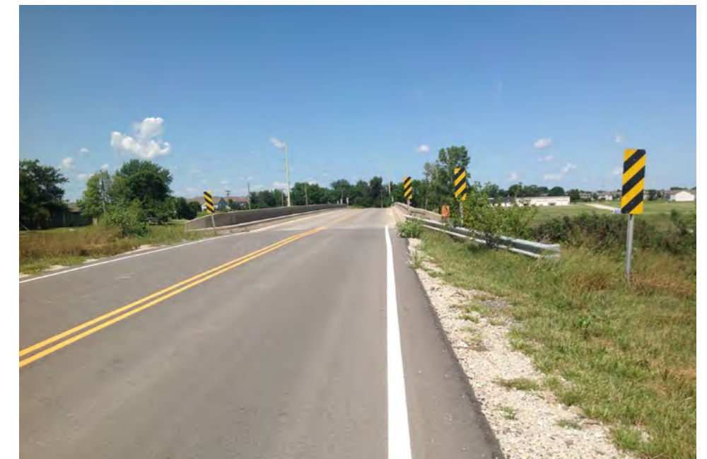
Moonlight Rd bridge over I-35. Photo: NPS
