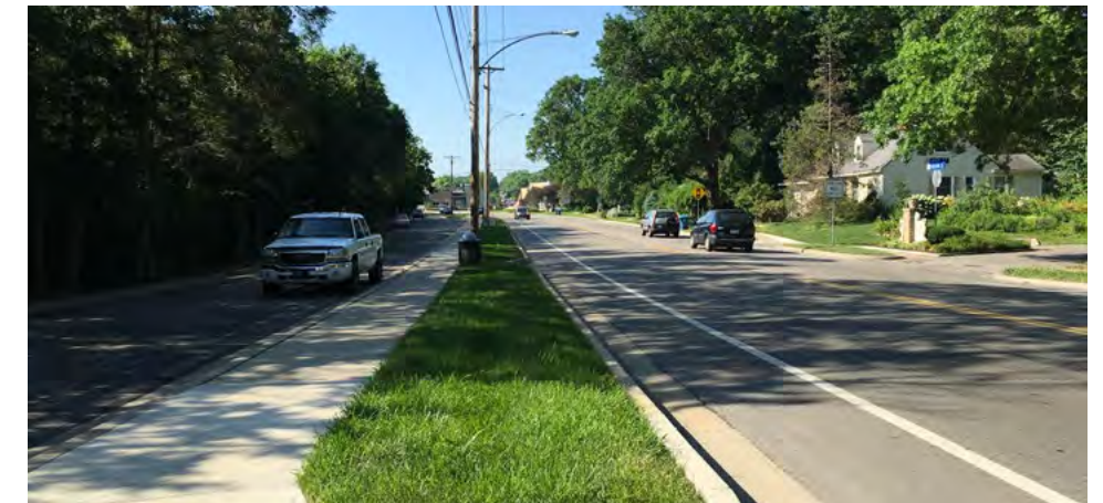
Mission Rd near W 68th St, looking south. Photo: NPS
