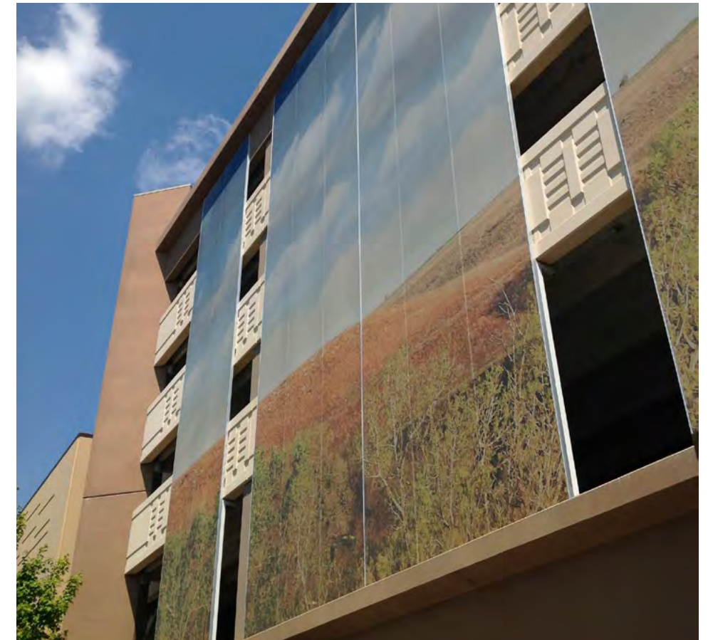
Large scale landscape imagery screens at the Prairie Fire Shopping and Entertainment Center, Overland Park, Kansas. These screens are translucent when viewed from inside the parking structure. Photo: NPS.
