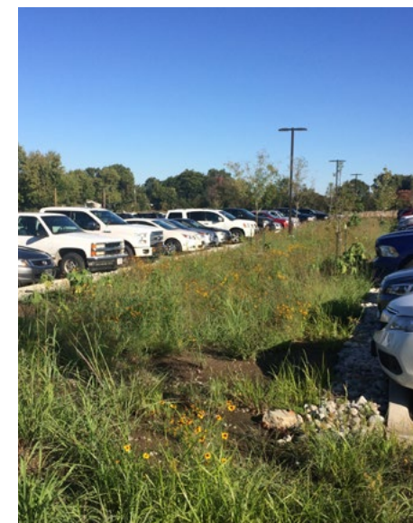
Bioswale feature at the CAA
