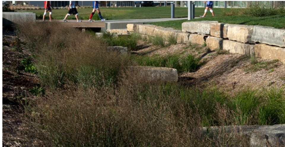
A bio-retention channel in Greensburg, Kansas utilizes a wide street right-of-way to capture and treat stormwater from the public street and high school property. A pedestrian bridge allows users to experience the green infrastructure as a design element.
