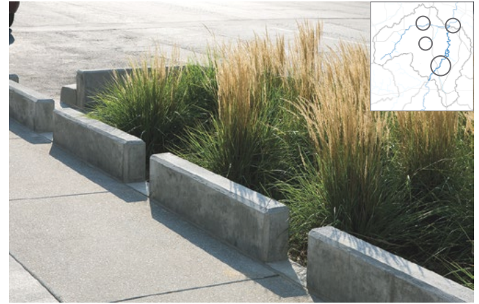
Urban & Suburban Street BMPs
