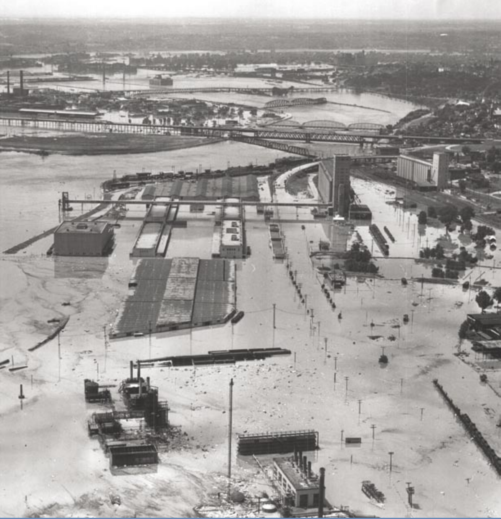
Aerial view looking south across the Fairfax District at the confluence of the Kansas and Missouri Rivers during the 1951 flood.
