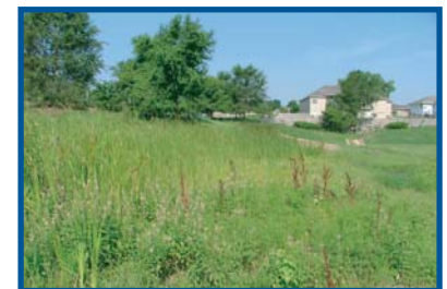
The sides of the detention basin were planted with native prairie wildflowers and grasses.
