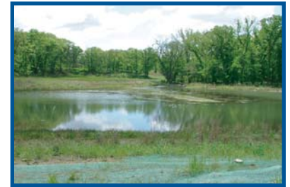
The infiltration field (in background) provides recreational space and quickly drains run-off into the wetland (in foreground).
