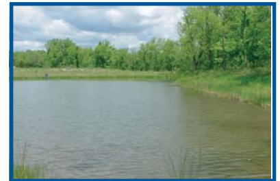
Western wetland treats stormwater prior to entering newly-constructed 33-acre Lake Lenexa (downstream, not pictured).
