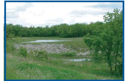
Wetland treats stormwater flow from Prairie Star Parkway (upstream).
