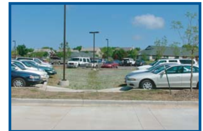
Stepped bioretention cells for filtering runoff from the parking lot.
