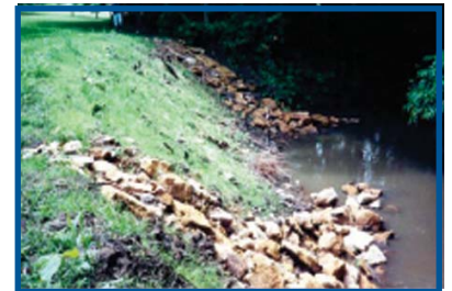
Example of using natural stabilization to divert and reduce the flow of water.
