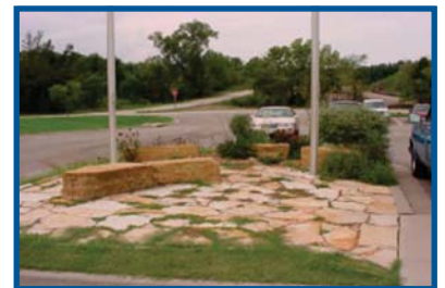
The flagstones provide a more pervious surface to improve infiltration of stormwater.
