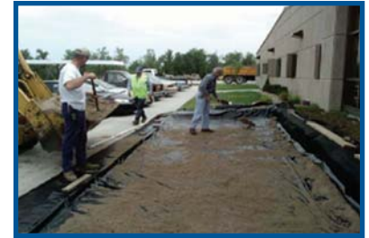
Construction of the roof drained rain garden.
