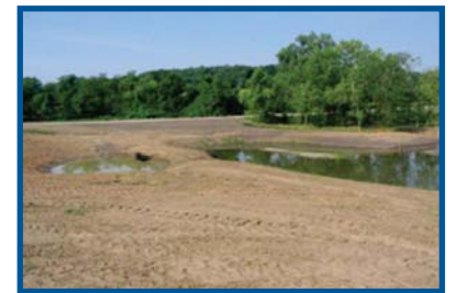
Sediment forebay provides some pretreatment of stormwater.
