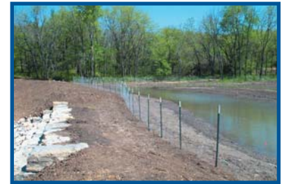
Animal fencing installed to keep the geese from eating the wetland plants.
