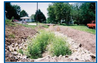
The finished bioretention swale immediately after construction.
