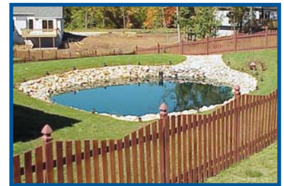
Stormwater retention basin.
