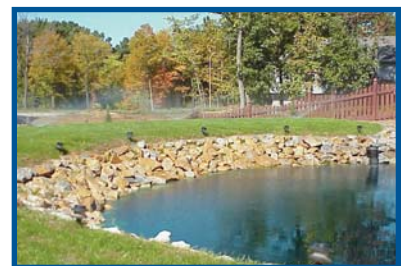
View of sprinkler system and its recycled water source.
