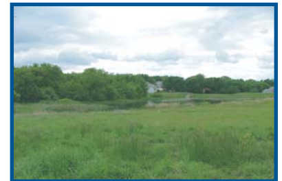
The joint-use stormwater treatment facility serves as a valuable community amenity.
