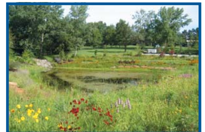
Wet pond with native plant edge treatments.
