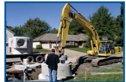
Installation of the Vortcapture VC-70.
