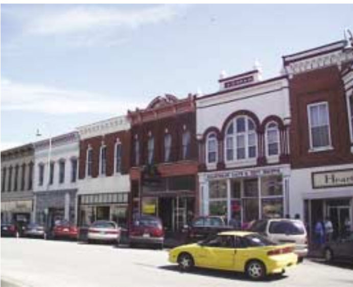
Highly articulated buildings such as these visually shorten perceived distances and encourage pedestrian activity.
