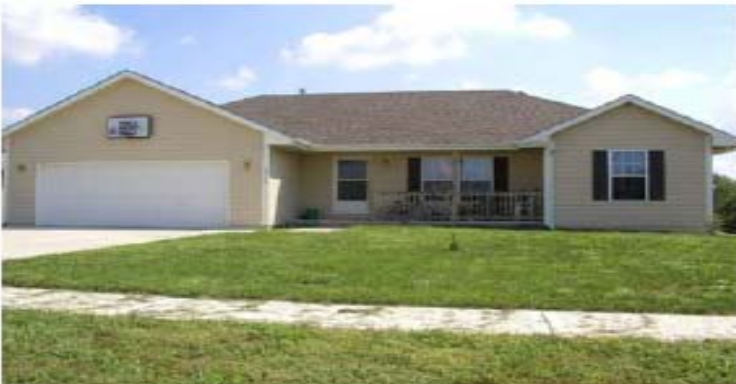
The porch is not raised 30" above the sidewalk.
