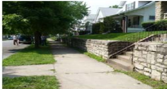
A retaining wall raised the lawn above the sidewalk.
