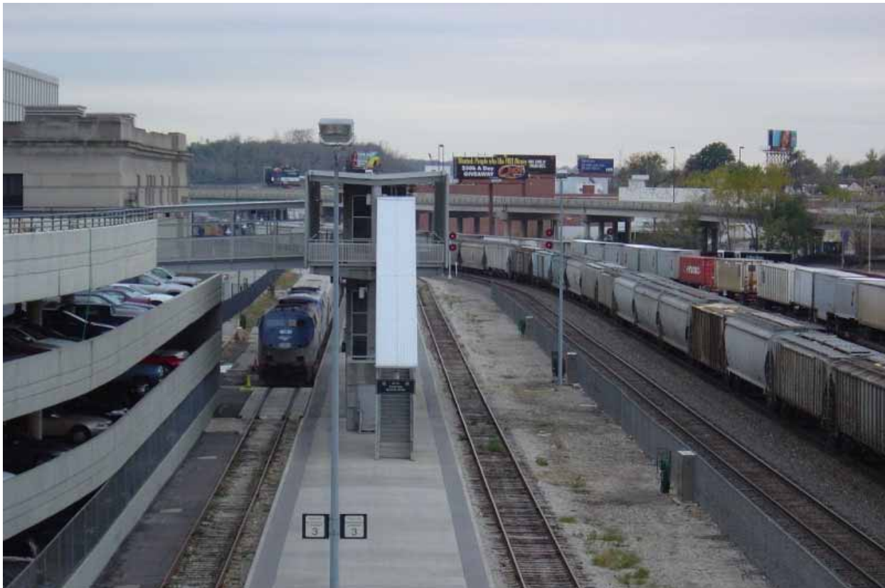
Figure 3.1 Union Station Passenger Rail Platform
