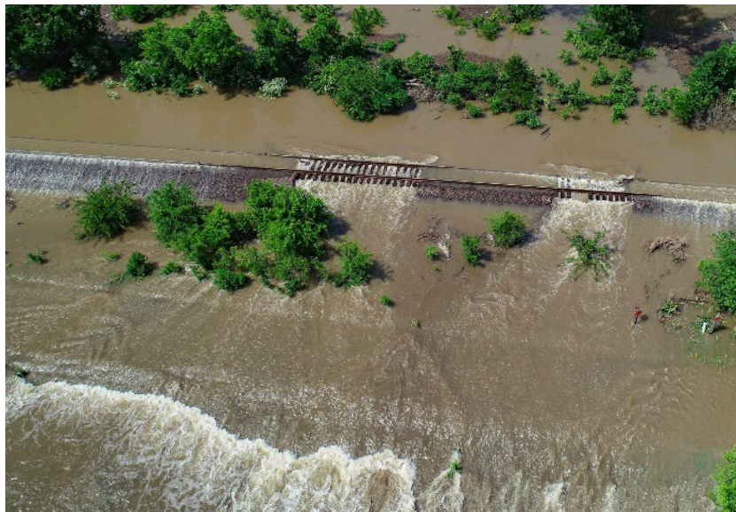
Figure 4.10.1: Breached Levee in Levasy, Missouri
