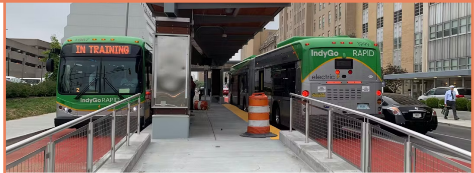
IndyGo BRT Stop, Indianapolis, IN
