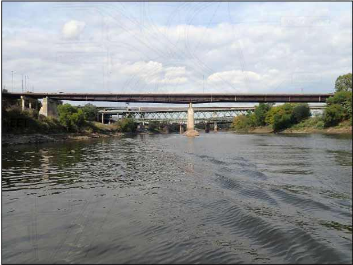
Photo 2 – Downstream (East) Elevation
