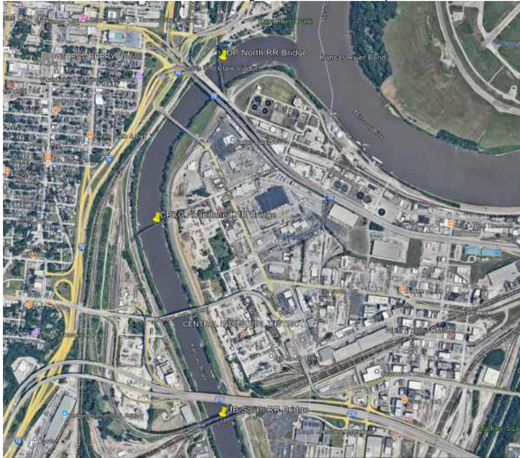
(RR Bridges in Study Area)
