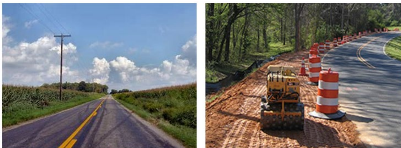
Figure 2. Typical Rural Street/Highway without Complete Streets Application (left) and Rural Highway with Widened Shoulder for Cycling (right)
