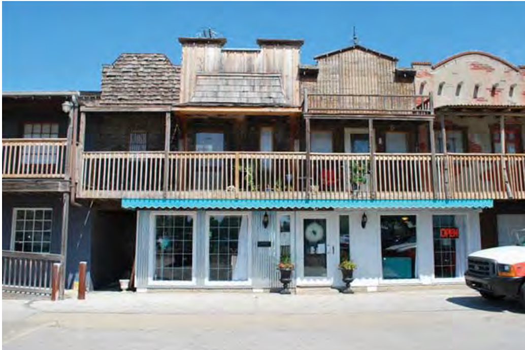
Fig. F.12 – An example of a highly complex storefront system added after the building was built. This storefront does not relate to the other structures within the downtown. (SRJA, 2013).
