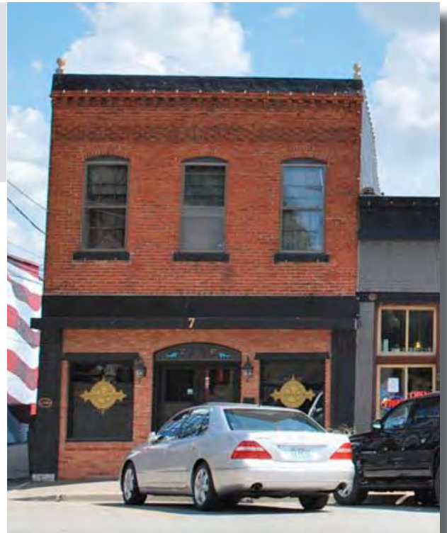
Fig. F.22 – Example of new wall sconce lighting located on either side of the main entry door on this restored building downtown. (SRJA, 2013).
