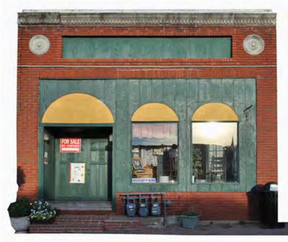
Fig. F.5 – View of an existing storefront in downtown Parkville. (SRJA, 2013).
