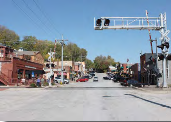
Fig. B.8 – View looking north down Main Street (SRJA, 2012)
