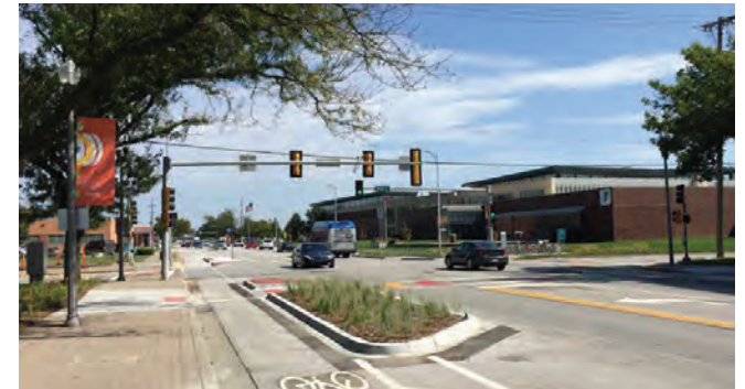
FIGURE 2.36 - ARMOUR ROAD BUFFERED BIKE LANES - NORTH KANSAS CITY
