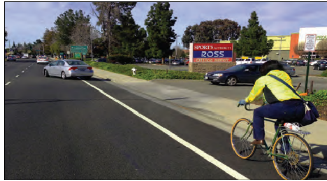
FIGURE 2.31 - UNPROTECTED BIKE LANES REPRESENT A LOW BICYCLE COMFORT FACILITY
