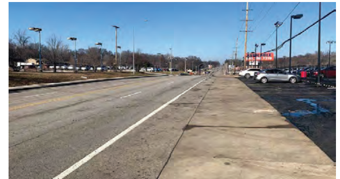
FIGURE 2.29 - SIDEWALKS AT THE SAME ELEVATION AS THE ROAD WITH NO SEPARATION, RESULT IN LOW WALKING COMFORT
