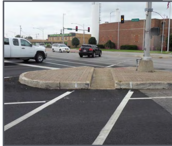
Figure 5.9: Crosswalk noncompliant with Americans with Disabilities Act (ADA) standards at Burlington Street and Armour
