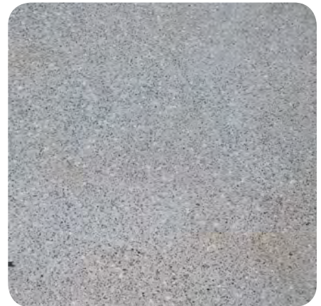
Image of concrete surface texture with concrete deactivator application
