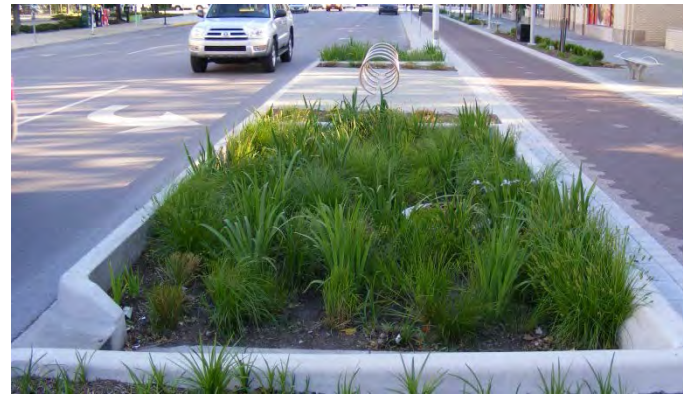
Figure 47: Infiltration planters treat and manage stormwater runoff.
