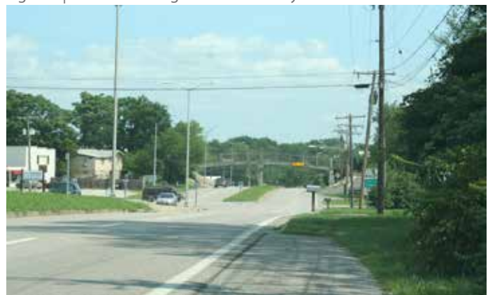
Figure 5 | Photo looking east at the pedestrian bridge.
