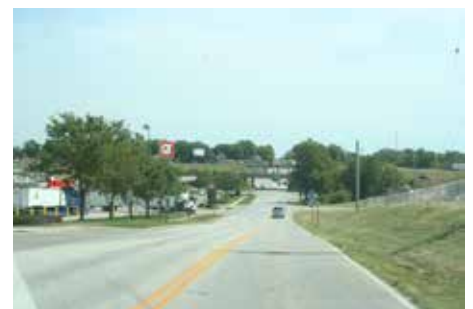
Figure 40 | Photos of existing road conditions in the corridor.
