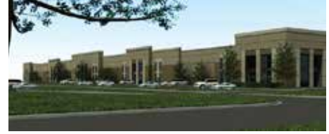
Figure 70 | An example of an industrial building.
