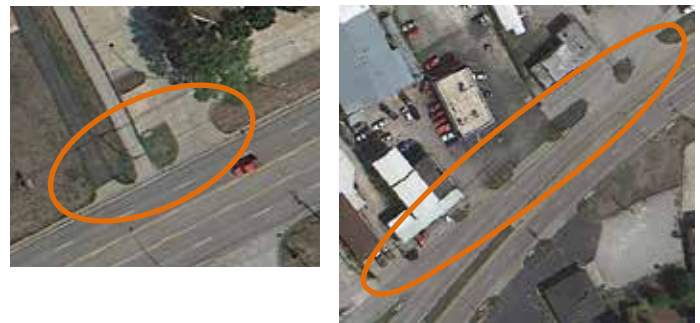
Figure 47 | These two images show examples of closely space driveways within the corridor.
