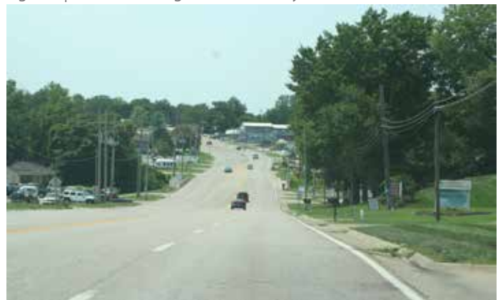
Figure 4 | Photo looking west from the Bryant Street intersection.
