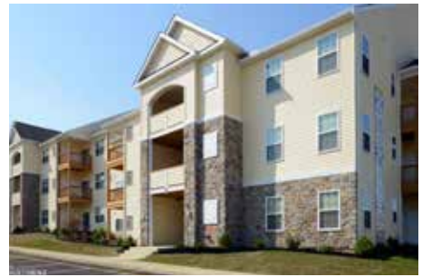
Figure 59 | Multi-Family apartments that could serve as workforce housing.
