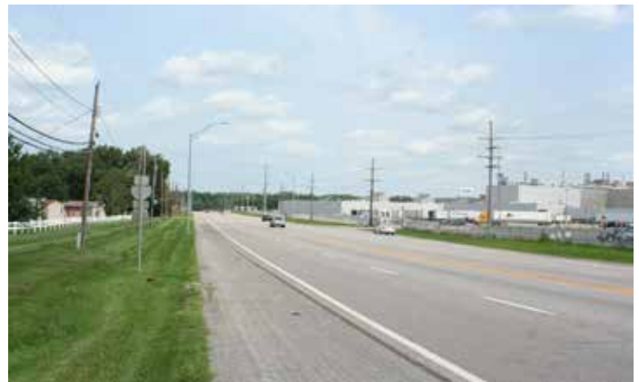
Figure 9 | Looking east near the Palmer Road intersection.
