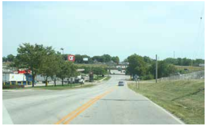
Figure 18 | Looking east from Sobbie Road.
