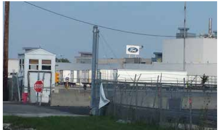
Figure 10 | Chain link fencing with barbed wire along the south side.
