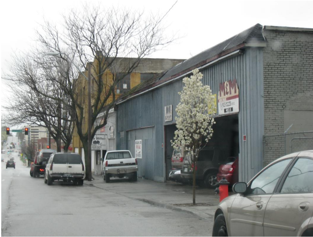
Former retail space reused as auto servicing at 4524 and 4528 Troost Avenue (Deteriorated or inadequate site improvements, Economic and social liability)
