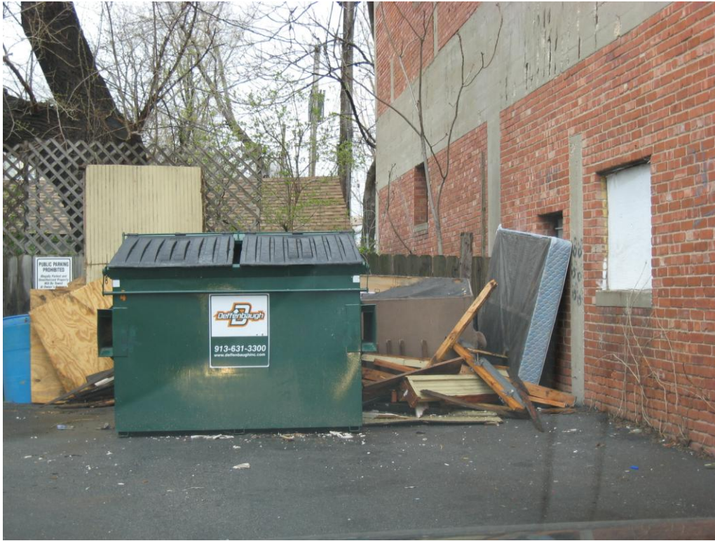
Unscreened trash disposal and debris on west side of 4538 Troost Avenue ( Unsanitary or unsafe conditions, Conditions which endanger life or property )
