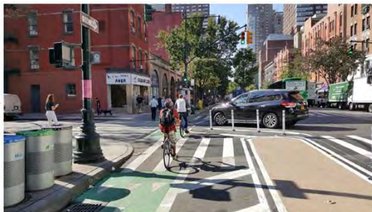
Figure 7-15: Corner Island with Flexible Delineator Posts (Source: Carl Sundstrom, PE, Office of Bicycle and Pedestrian Programs, New York City Department of Transportation)
