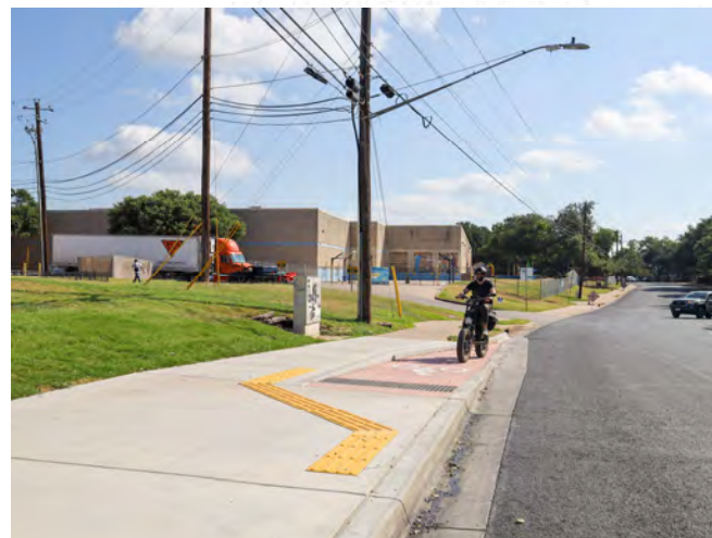
Detail 1—Preferred bicycle ramp alignment with wide sidewalk buffer
