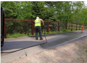
Figure 15-4: Fog Sealing a Shared Use Path
