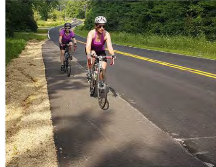
Figure 12-3: Shoulder Widening on Uphill Section of Roadway to Accommodate Bicycling
